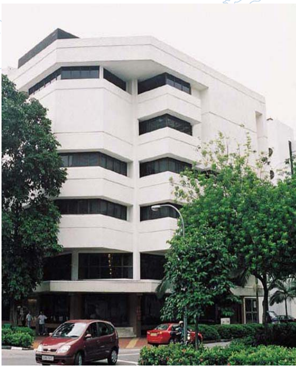
Before Refurbishment: a 6-storey office building
