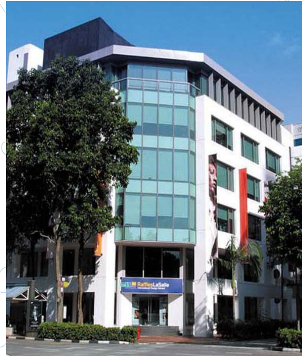
After Refurbishment: - more rentable area - new building facilities and M&E services
